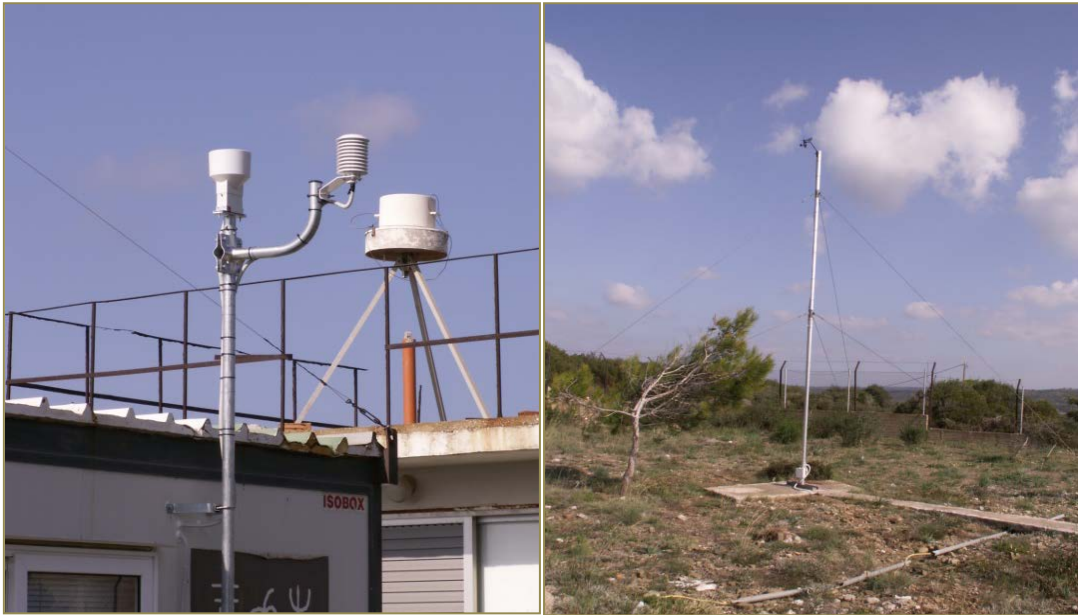
Figure 1: The new automatic meteorological station at Methoni
